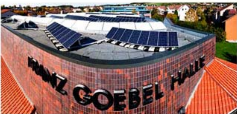
SWR - GH - Photovoltaik 005.jpg
