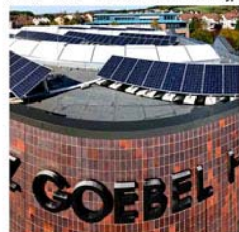
SWR - GH - Photovoltaik 006.jpg
