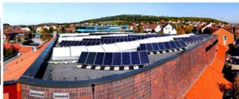
SWR - GH - Photovoltaik 002.jpg
